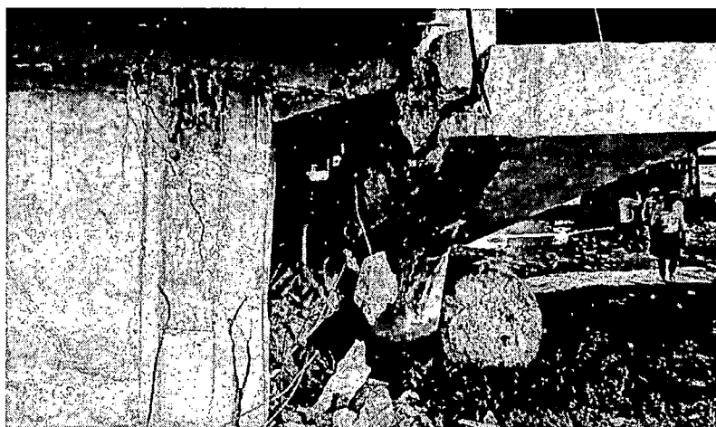
Plate-5: Damages of girders of dislodged span
