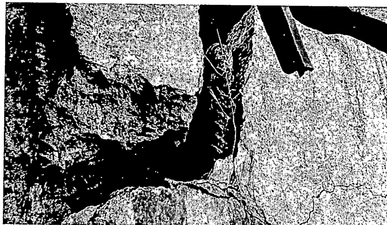
Plate-9: Lack of bond between concrete and bars of the pier cap
